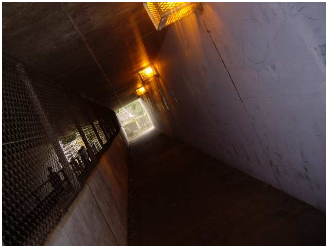
Picture 1: Fordoun Underpass Prior to Intervention
